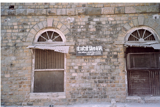
Arched door and window openings in coursed Malad / Kurla stone
