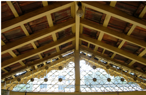
Timber roof with mangalore tiles
