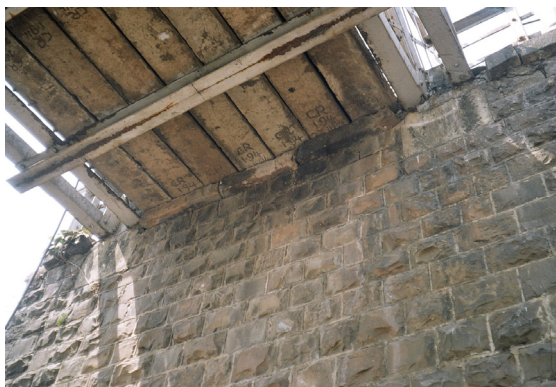
Coursed masonry wall supporting the floor
