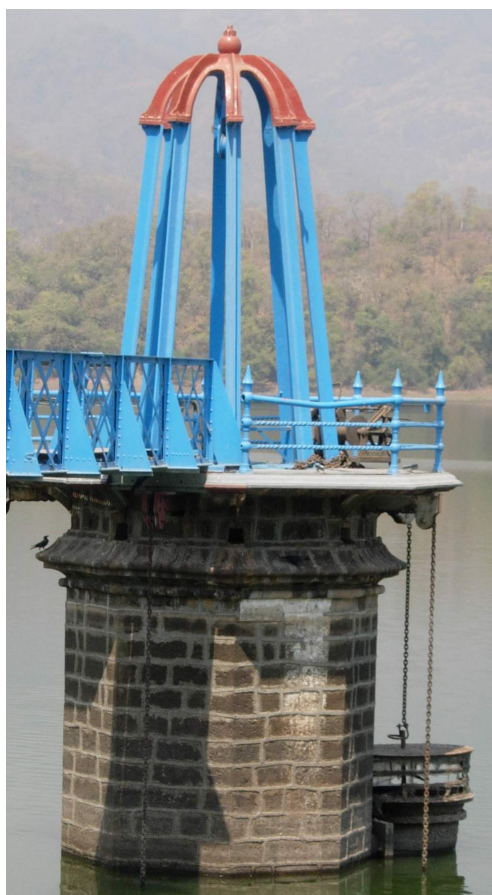
The outlet Tower with Plugs and Strainers
