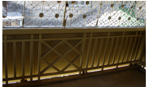
Wooden balcony railing with MS grill
