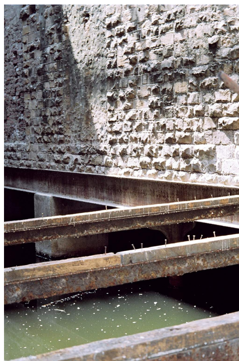
Water Tanks – an essential part of textile mills constructed in Stone, Structural Steel and RCC
