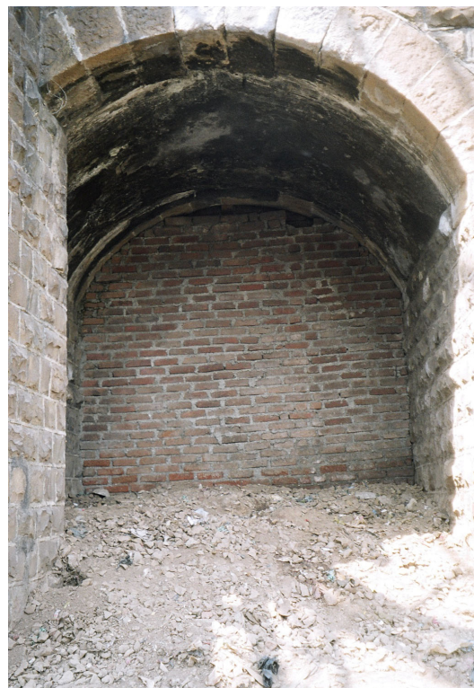
Road side of the arch closed in brick
