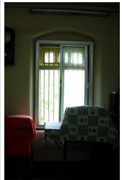
Aluminium sliding windows fixed internally without disturbing the existing wooden windows
