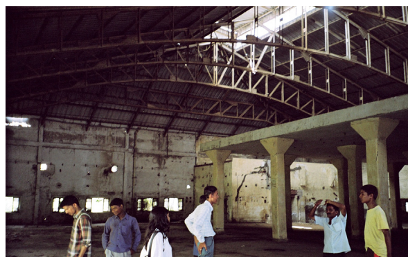
Roofing in structural steel covering large spans
