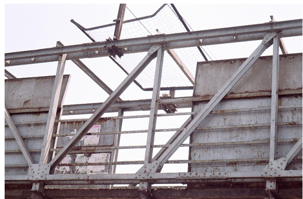
MS members forming the support system
