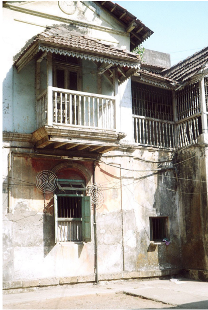
Wooden balcony with sloping roof supported on wooden joists
