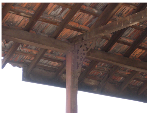
Iron brackets supporting the roof
