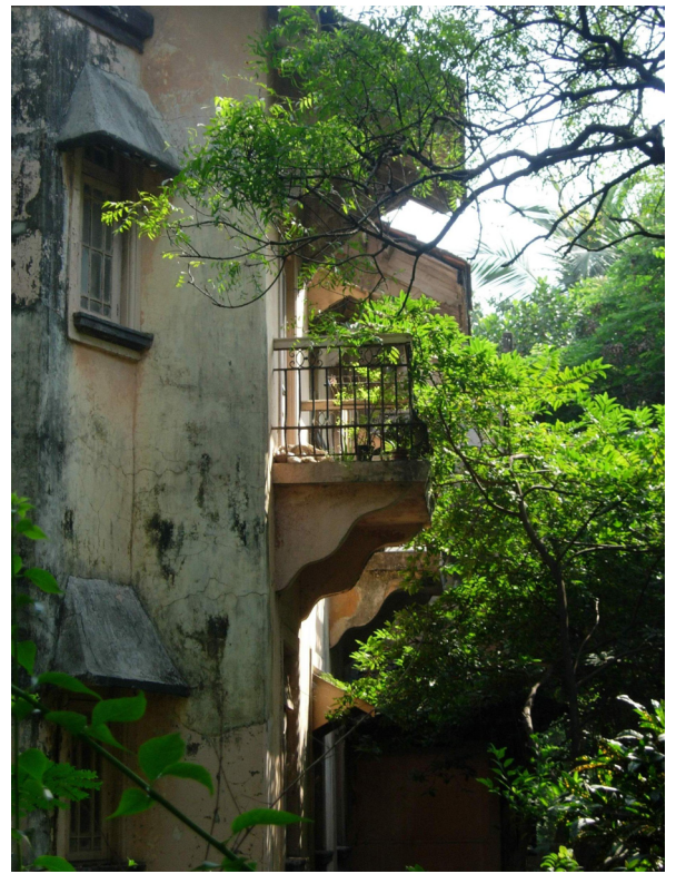
Concrete brackets supporting balconies
