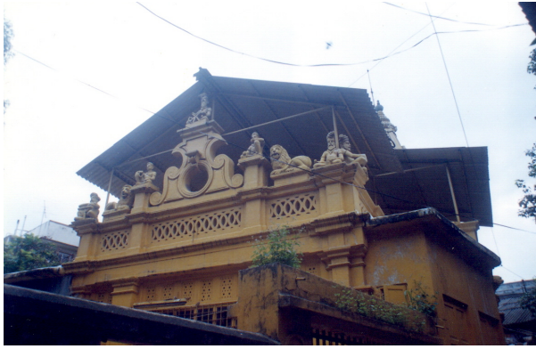
Addition of AC sheet sloping roof
