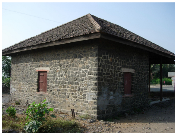
The structure in stone masonry
