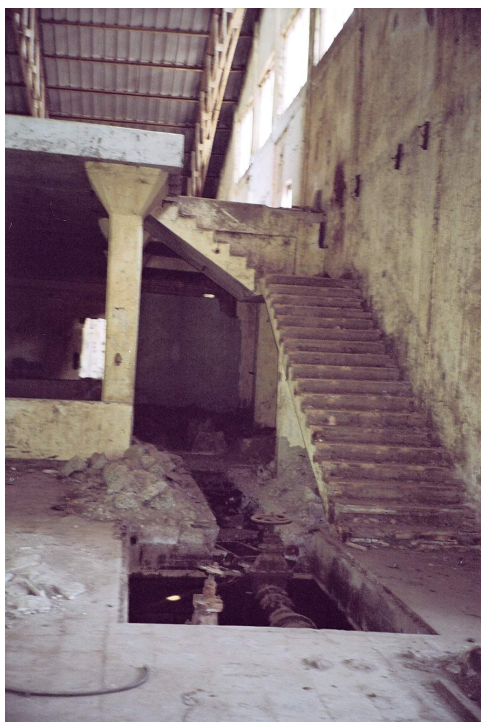
The RCC staircase connecting to a mezzanine level
