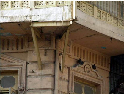
Balconies supported by MS sections
