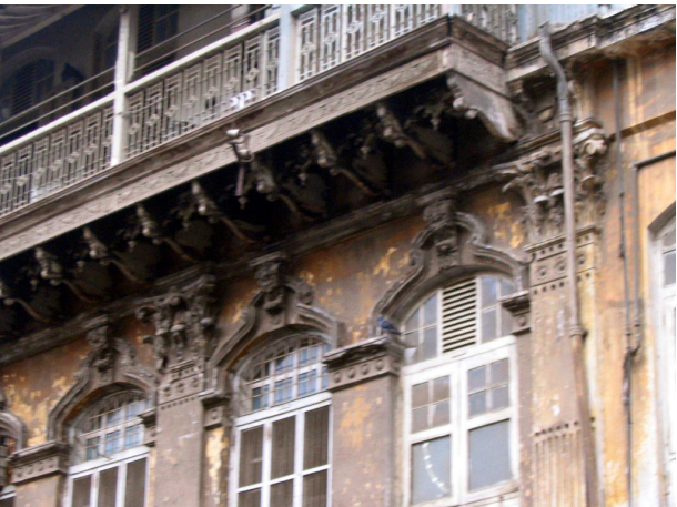
Decorative wooden brackets support the projecting balcony
