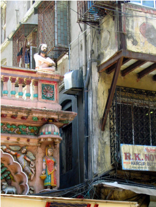
The services are housed in the 0.6m gap between the two buildings
