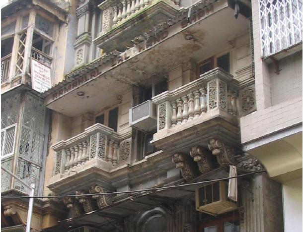
Decorative concrete balustrade and brackets for the projecting balconies
