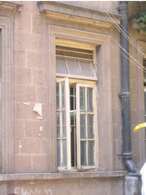
Simple architraves around the windows
