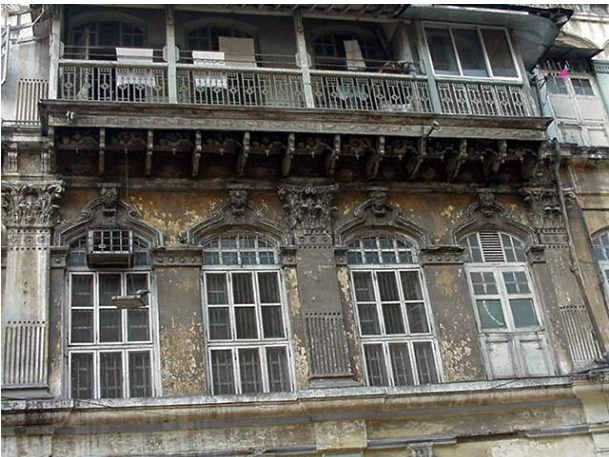
Segmental arched openings with decorative mouldings and key stones
