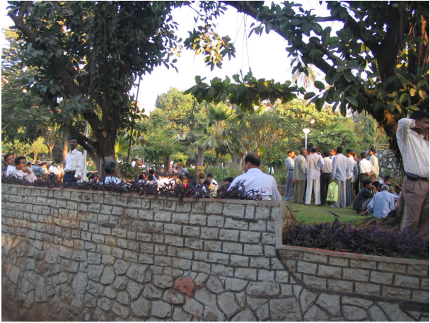
Combination of random rubble and coursed ashlar masonry retaining wall
