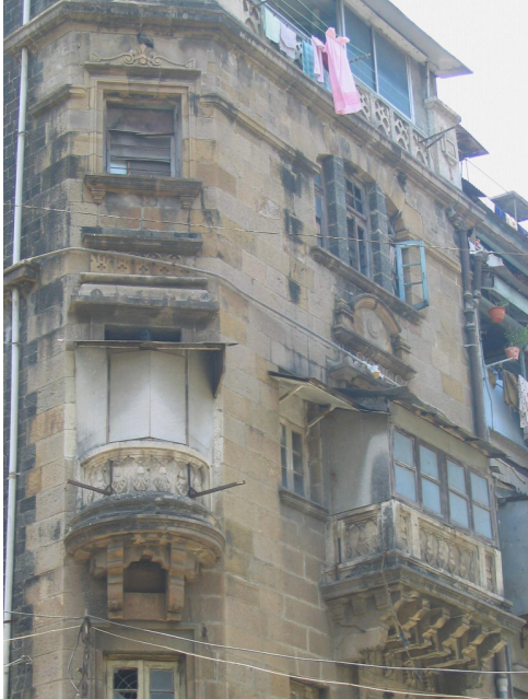
Projecting balconies supported by decorative brackets
