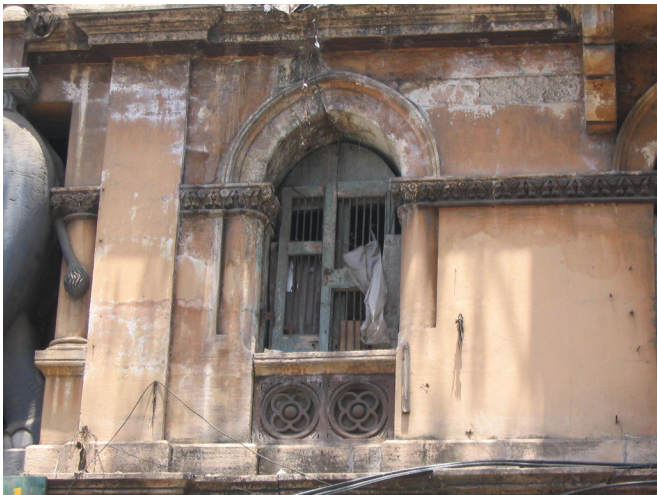
The wooden members of the windows need replacement
