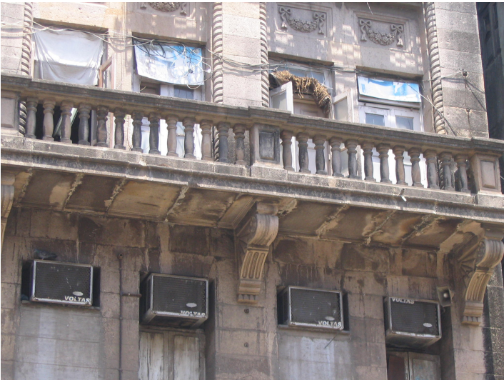
Window air-conditioning units below the projecting balconies supported by decorative brackets
