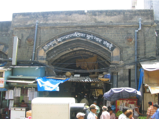
Black Basalt stone façade in coursed ashlar masonry
