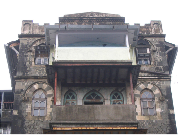
Projecting balcony reinforced later with M.S joists
