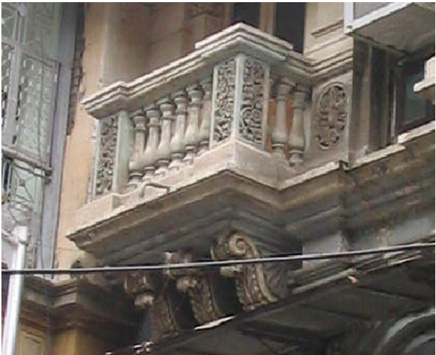
Decorative concrete balustrade and brackets for the projecting balconies
