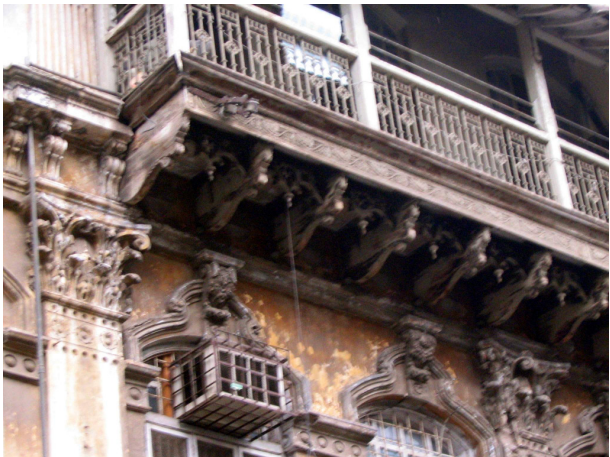
Decorative wooden brackets support the projecting balcony
