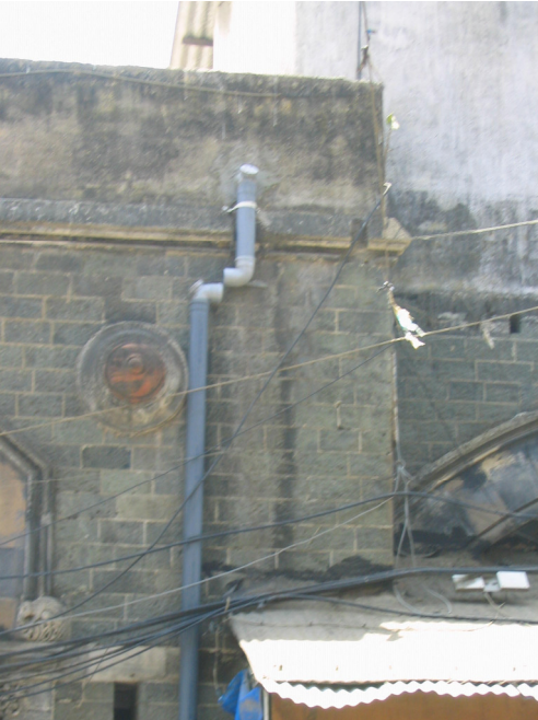
Black Basalt stone façade in coursed ashlar masonry
