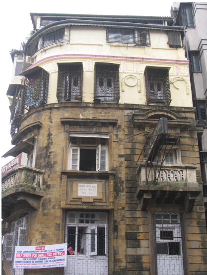
Malad stone cladded till the 3 rd floor
