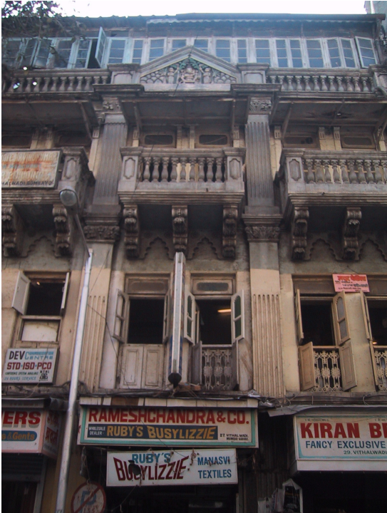
Fluted pilasters on the first floor and a decorative pediment on the third floor
