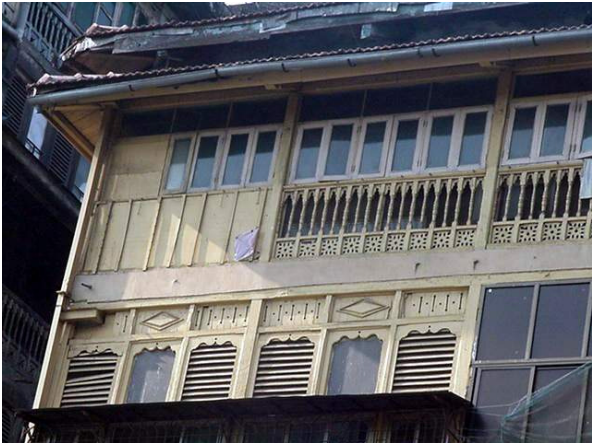
3 rd floor windows have been transformed to glazed folding windows
