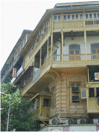
Balconies supported by MS sections
