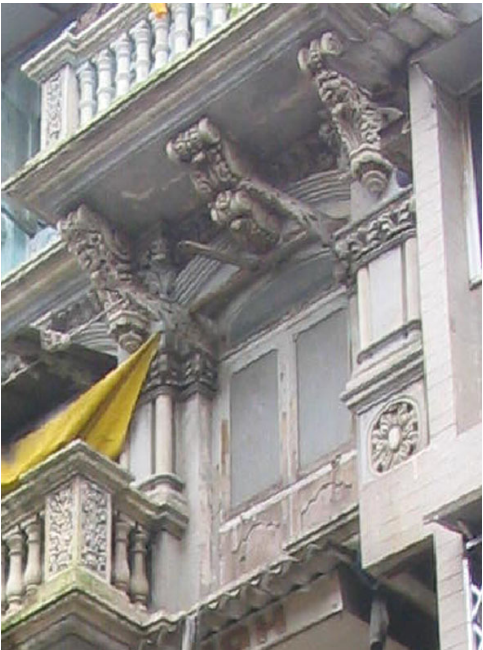
Highly ornamental brackets supporting the balconies
