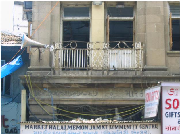
Electric cables hanging on the façade
