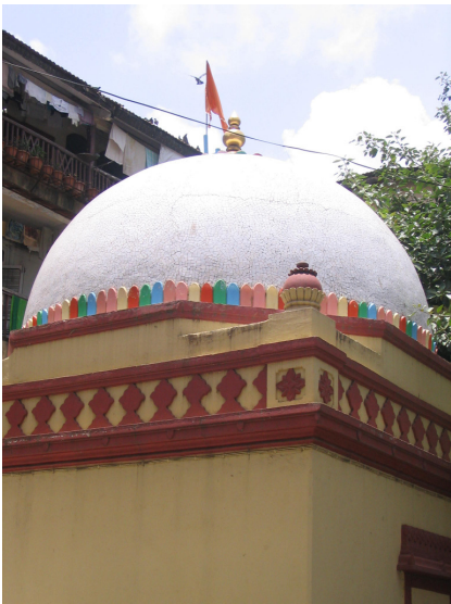
Dome is finished with China mosaic tiles
