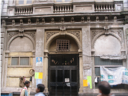
Semicircular arcade on the ground floor
