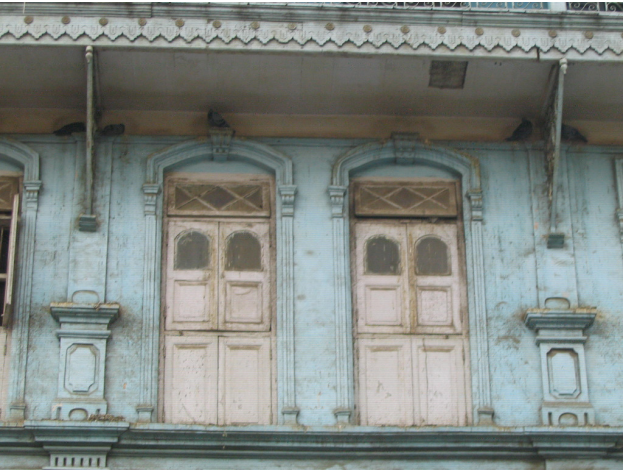
Windows are double height and the balcony above is supported by wooden brackets
