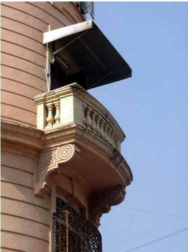
Projecting balcony supported by decorative brackets
