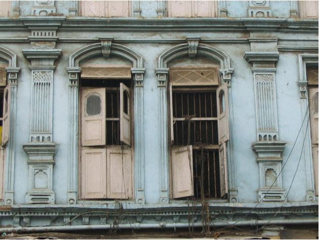
Decorative pilasters and architraves for the double shutter windows
