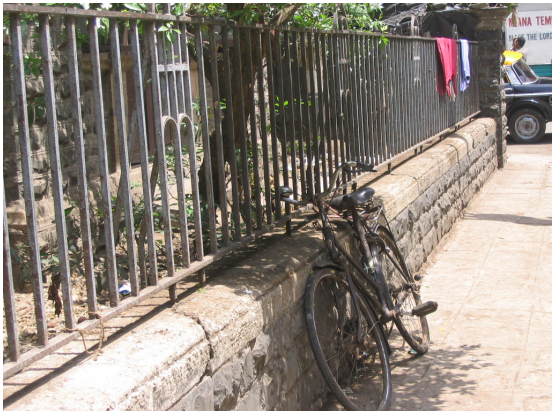
Black Basalt stone in coursed ashlar masonry compound wall with MS fencing
