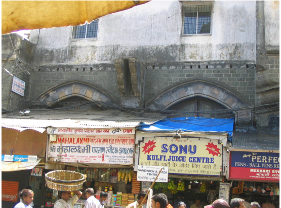
ashlar masonry seen only on the ground floor
