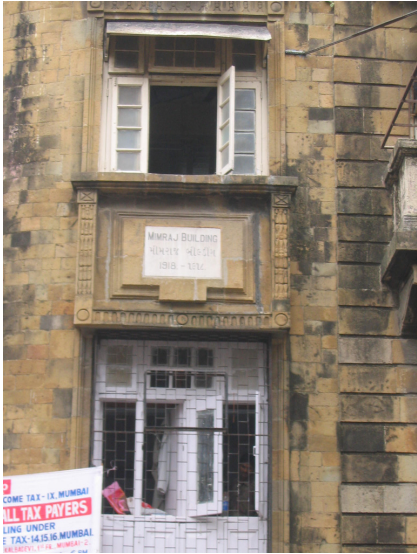
Coursed ashlar masonry on the façade
