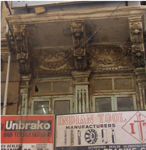
Detail of the balcony supported on the carved brackets
