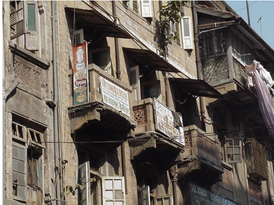
Detail of the balconies on concrete brackets with jali parapets
