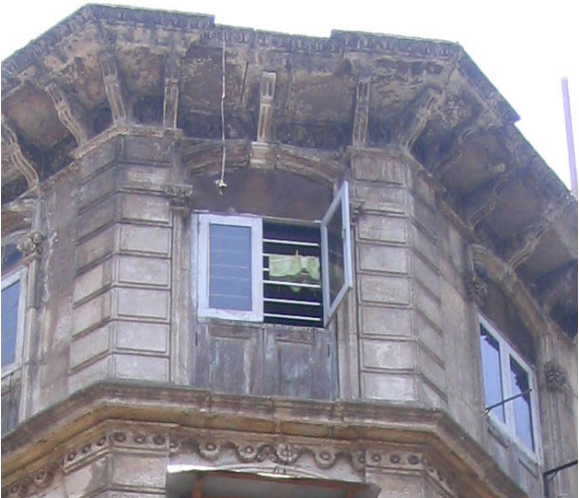
Detail of the projecting slab on brackets on the top floor
