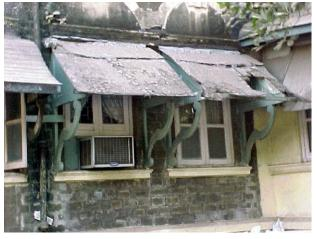
Sloping roof chajjas supported by decorative wooden brackets in poor condition
