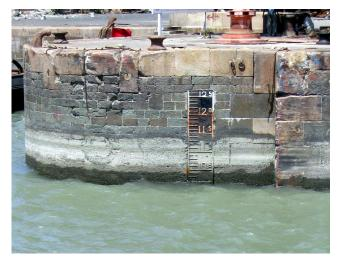
Indicator of the water level with markings on wall
